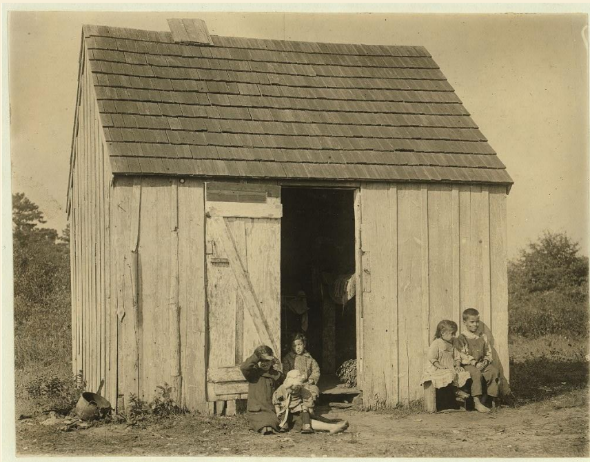
Small shack on Forsythe's Bog, occupied by De Marco family, 10 in the family living in this one room. Room is 10 ft. x 11 ft. x 5 1/2 ft. high and gable attic above. (See family picking cranberries in photo #1151.) Wooden toilets near at hand and bushes used as such, gave forth offensive odors. Turkeytown, near Pemberton, N.J. E.F. Brown Witness. Location: Pemberton, New Jersey. https://www.loc.gov/pictures/collection/nclc/item/2018674124
