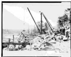
Title: 226. Early construction on section 2-A-1. This was the site of the first construction on the Blue Ride Parkway. - Blue Ridge Parkway, Between Shenandoah National Park & Great Smoky Mountains, Asheville, Buncombe County, NC
